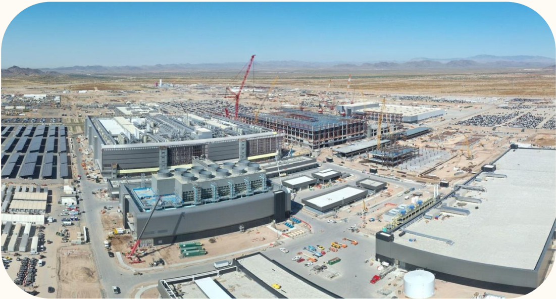
TSMC Arizona semiconductor manufacturing plant, opening 2025
