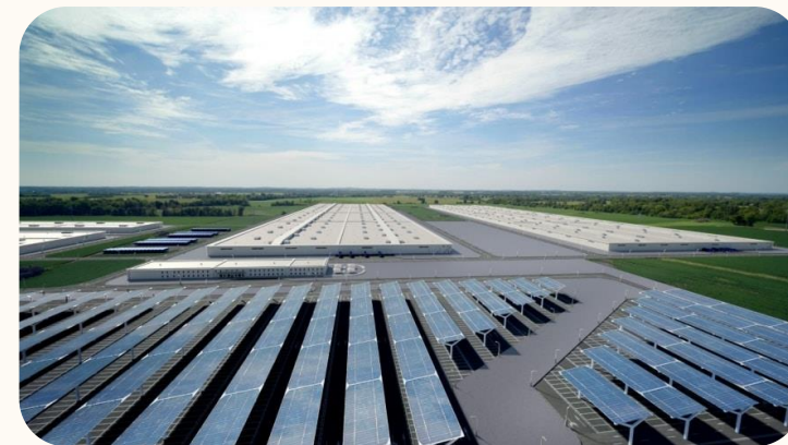
Ford / SK Battery Plant
